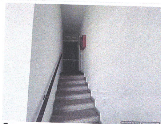
6 Stepenice do mansarde
